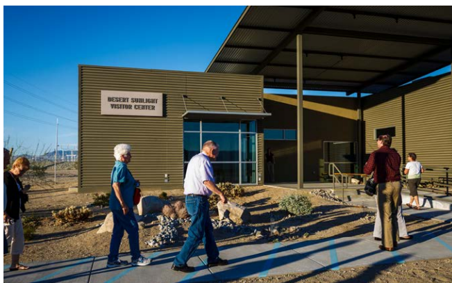
The Desert Sunlight Visitor Center provides an onsite solar learning center for students and the general public
