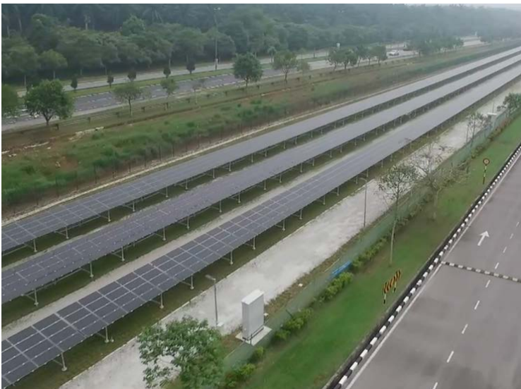
750 kW AC PV Installation at First Solar's Manufacturing Facility in Kulim, Malaysia.
